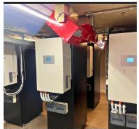
HARRINGTON STR, CAPE TOWN 300kW Deye HV with 360kWh Deye HV Lithium 2024
