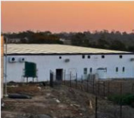
PETROSTOP, EAST LONDON 360kWp Solar PV Grid-Tie with 4x100kW Goodwe 2024
