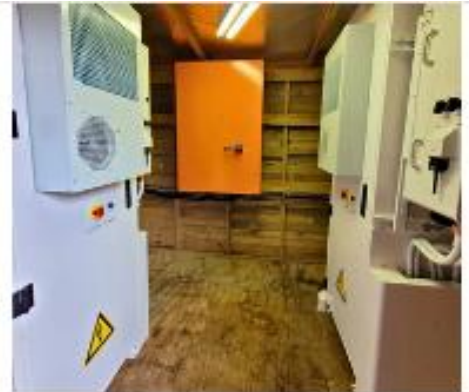
SKY VILLA, PLETTENBERG BAY 100kW Deye HV with 120kWh Sunwoda HV Lithium 2024
