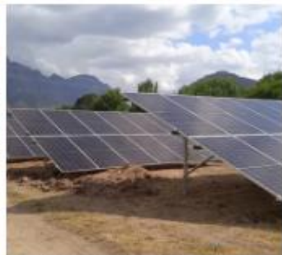
AUBERGE CLERMONT, FRANSCHOEK 24kWp Ground-Mount with 36kW Sunsynk and 70kWh Revov 2022
