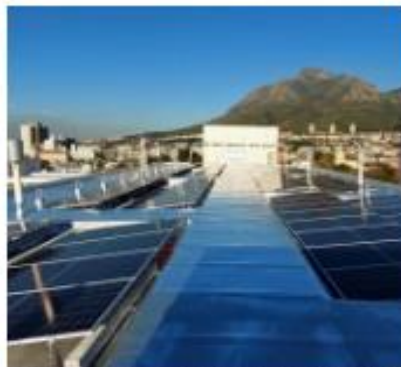
ST MARTINI GARDENS, CAPE TOWN 56kWp with 48kW Sunsynk & 246kWh Revov Lithium 2023
