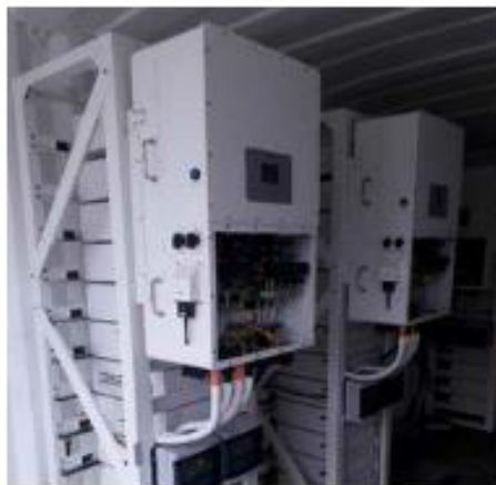
BUNGLAOW, PLETTENBERG BAY 150kW Deye HV with 184.3kWh Sunwoda HV Lithium 2024
